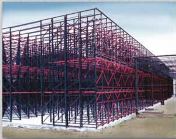
Rack Supported Buildings
